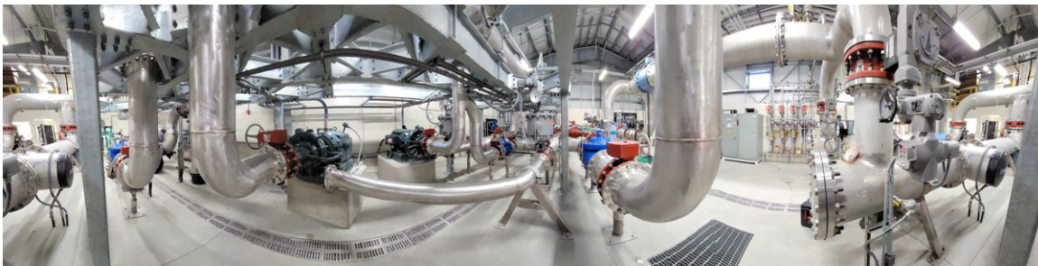
Photo 2: Dual F2W Installation
