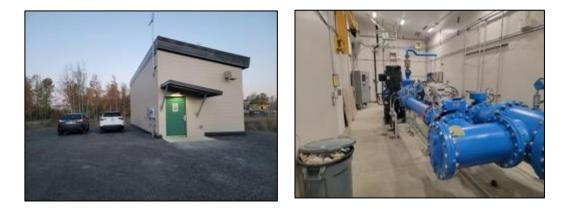
The first <u>AWWU deployment</u> includes a 40-kilowatt Rentricity NSF/ANSI/CAN 61 &372 certified Cornell pump-as-turbine unit within the City's water distribution system located in an above ground
