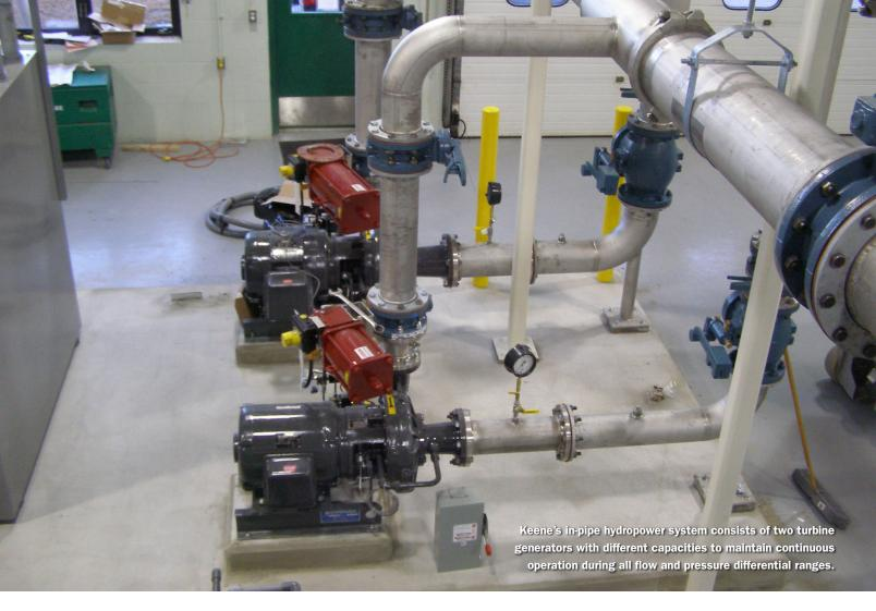
power system in parallel to the existing PRV inside the plant. Because of significant diurnal flow ranges, the in-pipe hydropower system consists of two turbine generators with different capacities to maintain continuous operation during all flow and pressure differential ranges. The in-pipe hydropower system also consists of associated electrical controls and water process controls.
