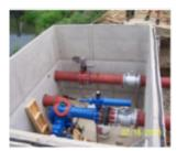
an insertion flow meter interfaced with the SCADA system.
