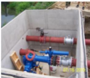
The mandated discharge system was adjacent to, but functionally separate from, the Beaver Run Raw Water Pump Station that provided raw water to the treatment plant on the adjacent hill.
